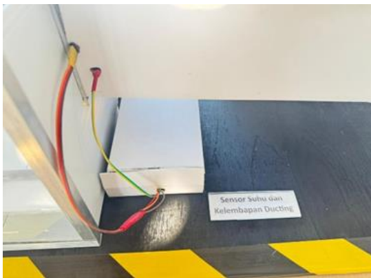
Picture 3. Placement of the sensor near the AHU ducting
